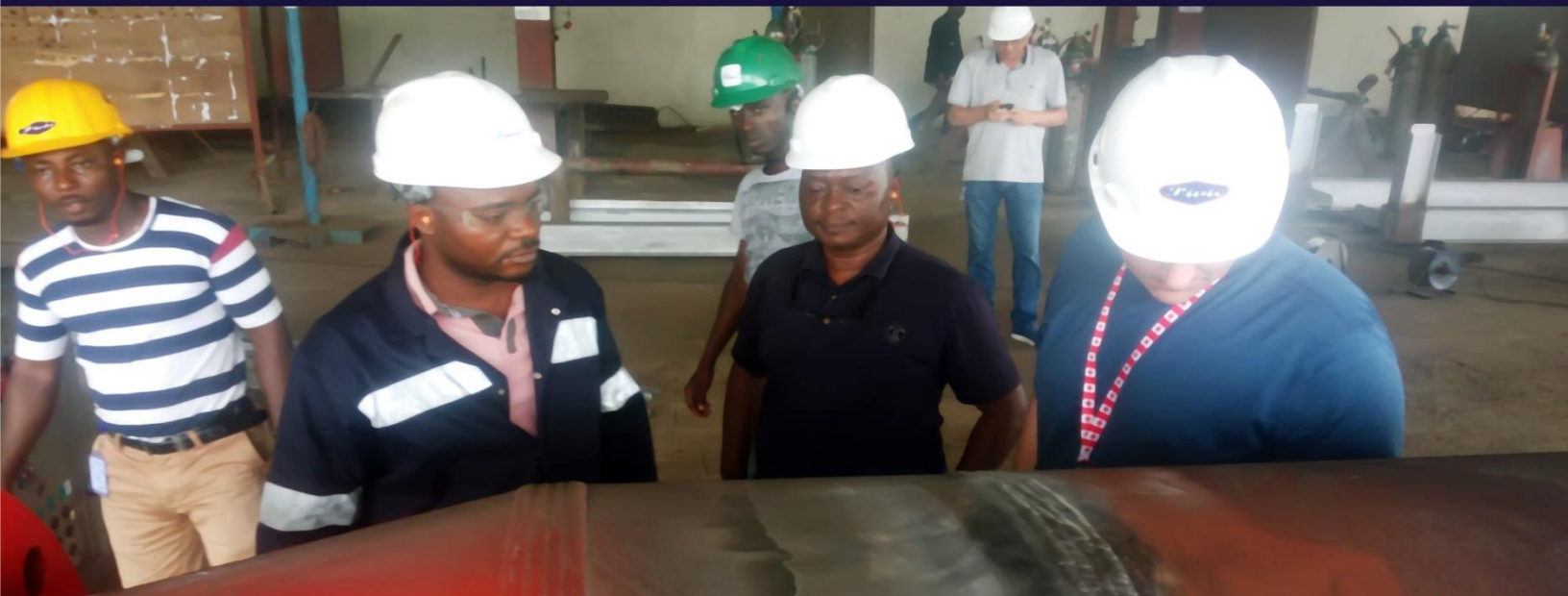
INSPECTION OF FABRICATED 30INCH PIPE
